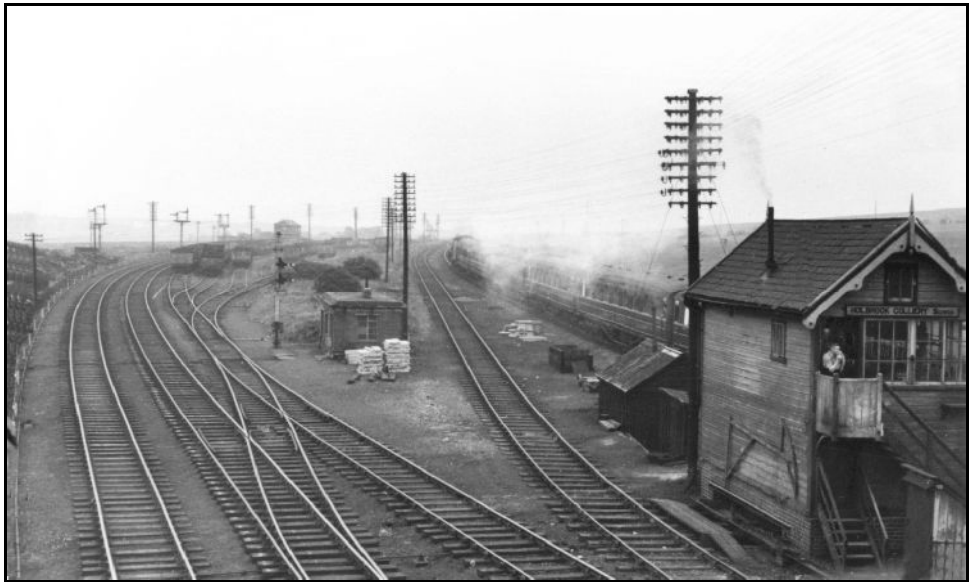
The view south from a footbridge south of Beighton station. Holbrook Colliery Sidings signal box is on the right with an up passenger on the former GC main line. The two lines on the extreme left are the original 'branch' from Woodhouse Junction to Beighton Jct on the 'Old Road' of the Midland. The Beighton Jct signal box is visible in the distance. Holbrook Colliery sidings, the site of the Cutting of the first Sod, were on the down side of the GC line to the right of the train in the photo, and close to the village of Beighton. All that remains today is the double track between Woodhouse Jct and Beighton Jct. photo: Jim Thompson collection
