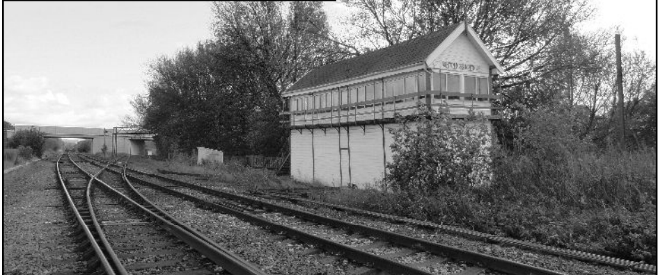
The tubular OHL stanchion seen at Ashton Moss North Junction photos: Chris Booth
