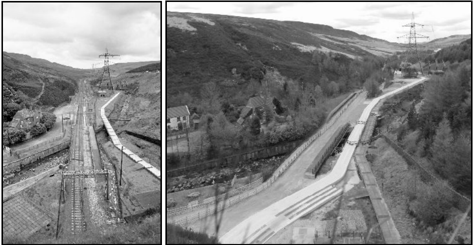
The view from above the Woodhead tunnels looking down Longdendale. left: Just a single track remains through the 'new' tunnel as track lifting nears completion in August 1986. The cable duct on the right connects the 'old' north tunnel to the electricity pylon.
