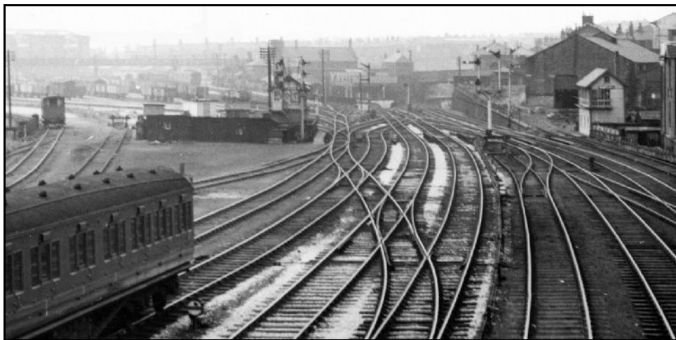
Looking west towards Oldham (Clegg Street) station (on the left) and Oldham Central (on the right). The two signal boxes are Waterloo Sidings (on the left) controlling the OA&GB lines and Oldham Mumps No.1 (on the right) controlling the L&Y lines. Waterloo Street passes under all these lines just this side of the signal boxes. Behind the photographer is Oldham Mumps on the L&Y lines and Glodwick Road on the OA&GB. All that's left today is the temporary Metro tram line to Mumps.
